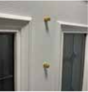
Visible fixings on the internal face – Hive knocker only.
